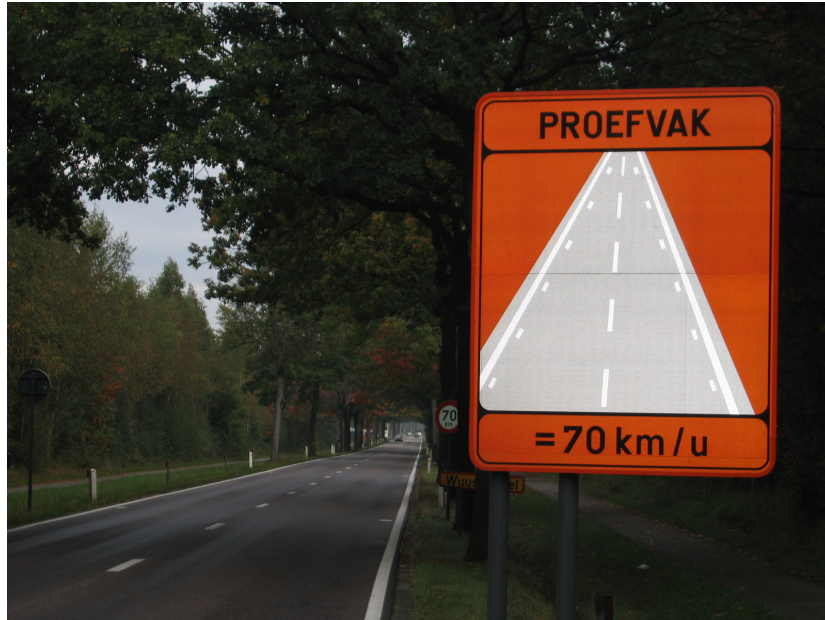
Figure 2: Line markings and information panel
